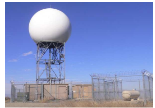
Weather Radar facility
